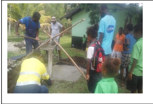
Pouring of concrete slab
