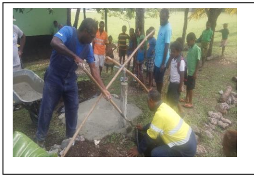
Pouring of concrete slab
