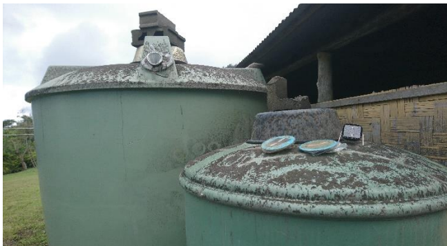
Gutters disconnected from tanks due to ash fall
